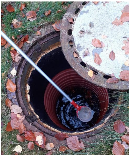
Figure 1: Top view of the rainwater utilization installation. Built underground are collection tanks for 200m 3 of rainwater (© T. Dorsch)
