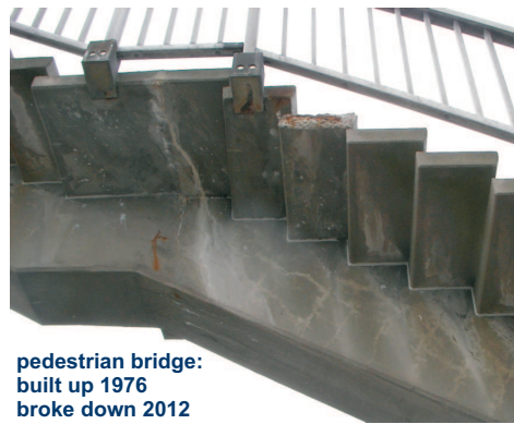
Fig. 1: Alkali-silica reaction (asr) in concrete causes cracks and loss of durability.
